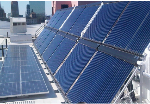
A typical rooftop solar thermal installation, one of several arrays, shown with optional PV
